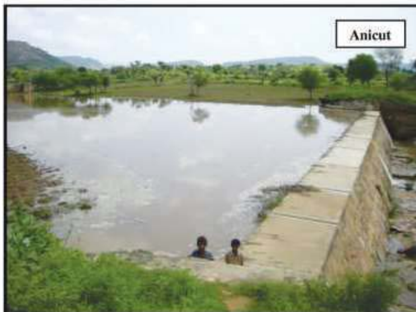
Groundwater recharge structure leading to percolation and soil conservation
